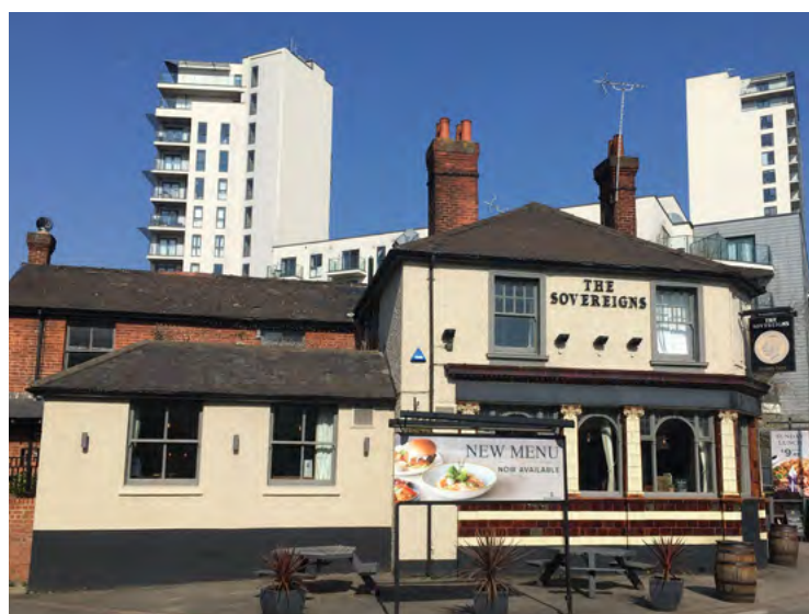
Fig 111 Sovereigns Public House from the south
