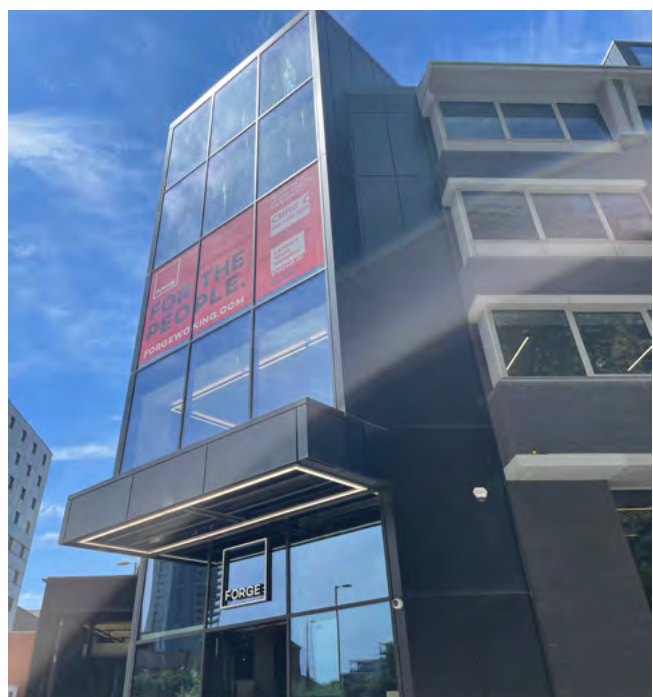
Fig 130 The Forge: Recently refurbished office
