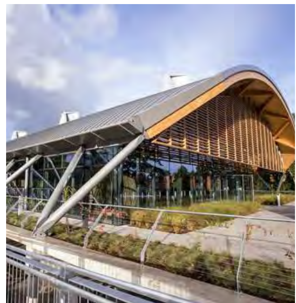
Fig 102 All timber used
