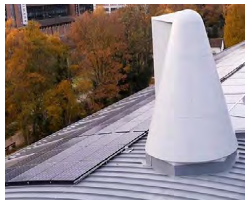
Fig 99 Passive ventilation and solar PV at the Living Planet Centre
