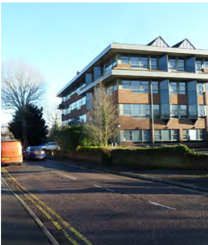
Fig 26 Photographs of the existing area condition
