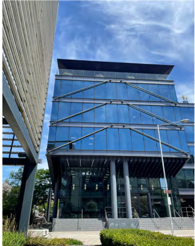
Fig 119 Recently refurbished McLaren office
