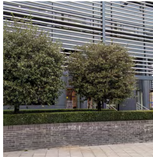
Fig 98 Brise soleil to reduce passive cooling and overheating
