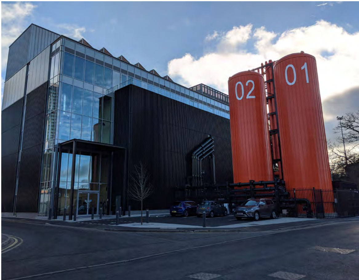
Fig 96 Combined Heat and Power Centre, Poole Road
