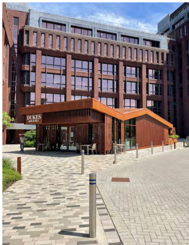
Fig 120 Dukes Court Offices in background with Deli in front
