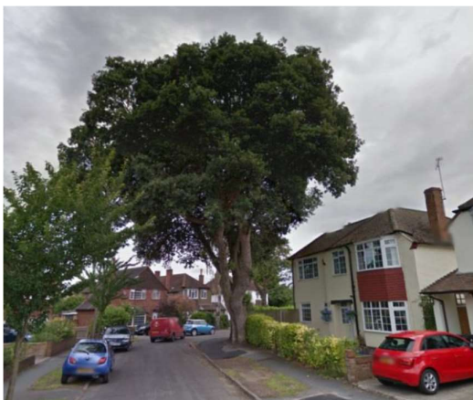
(2) Unsatisfactory distances between buildings and trees can cause overshadowing problems and root damage.
