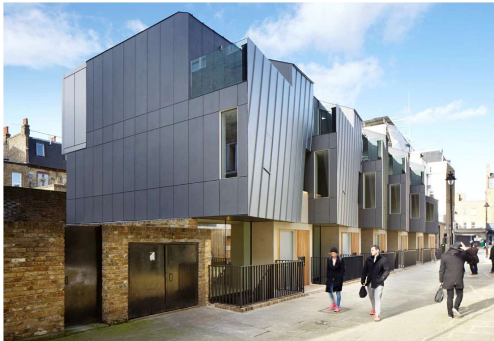
(15) Use of a controlled aspect design to avoid overlooking of adjacent dwellings - Example from Godson Street, London (Edgley Design)
