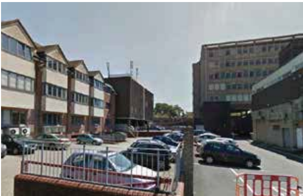
Prominent servicing/parking areas create poor quality streets
