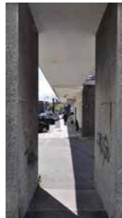
Run down built form
