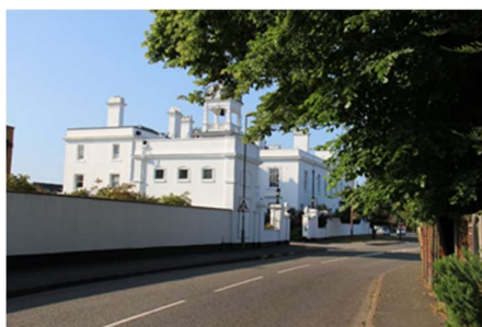
Figure 40 - The Clock HouseByfleet Mill (Grade II)
