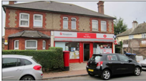
Figure 16 - Byfleet Post Office
