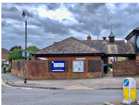
Figure 44 - St. Mary's Centre for the Community
