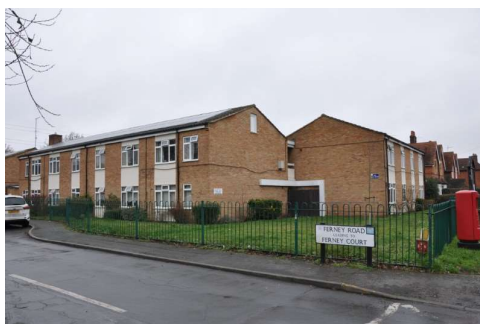
Figure 20 - Ferney Court supported accommodated
