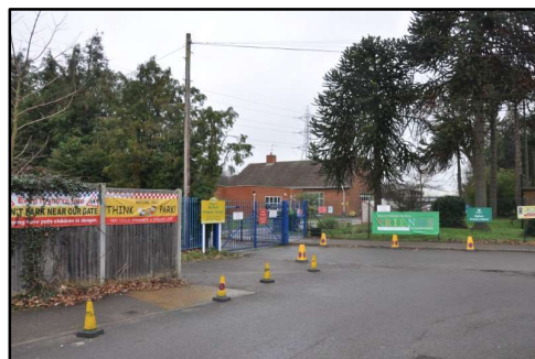
Figure 25 - Byfleet Primary School
