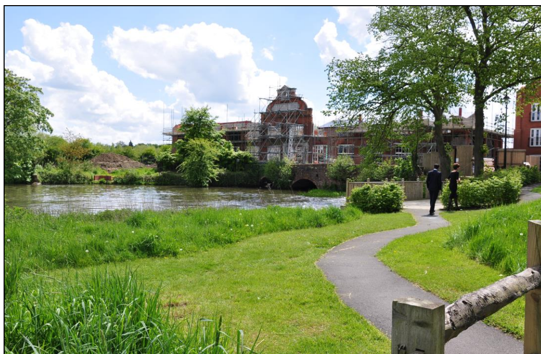
Gresham Mill, Old Woking
