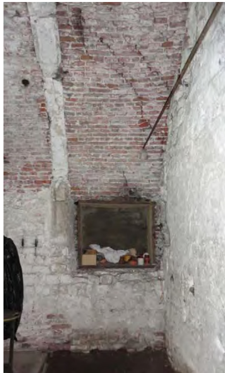
Figure 2. Cracking through brick vaults in bay 6 caused by insertion of window without lintel in 1920's.
