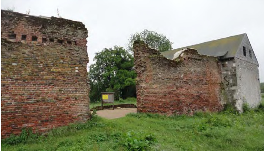
Figure 17. West Elevation of Service Building Wall remains showing unsightly white cement mortar capping to wall head and dampness concentrated at wall head due to rainwater run-off.
