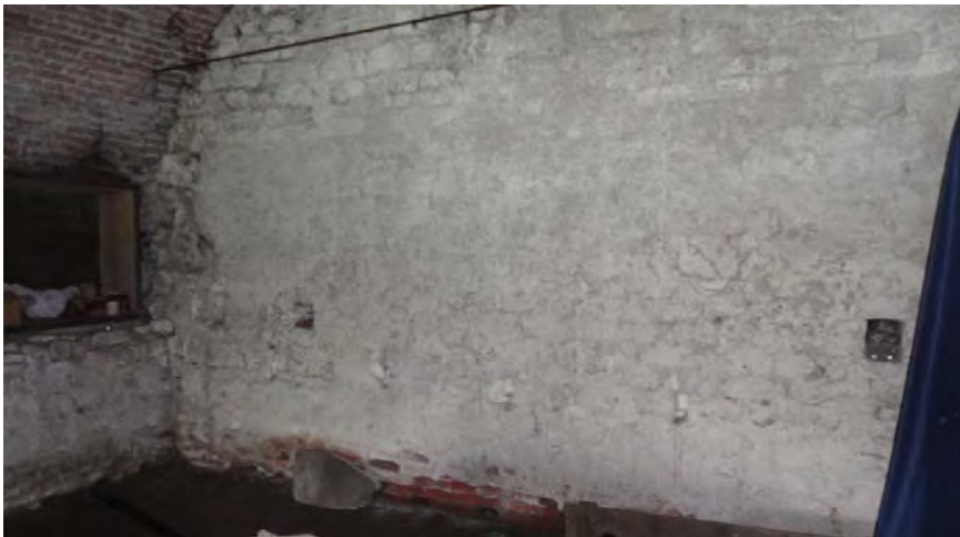
Figure 6. Lime Slurry coat and brick plinth to West Gable.
