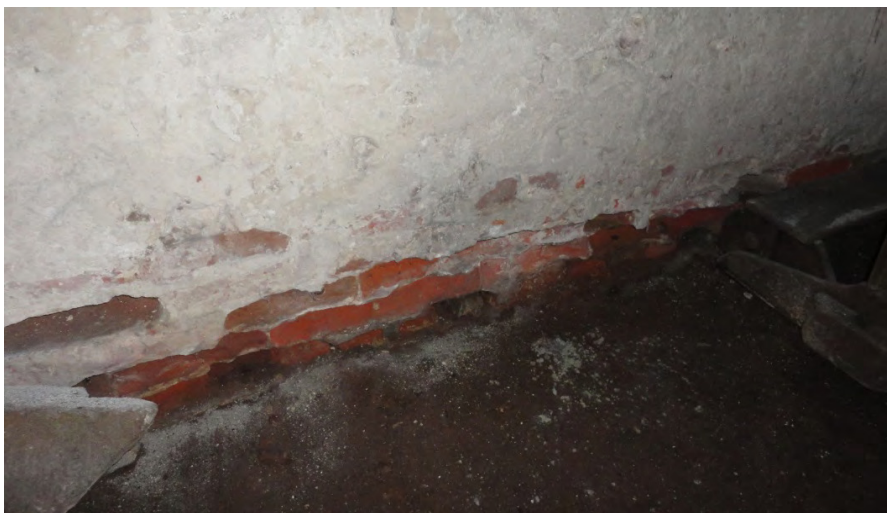
Figure 4. Eroding bricks to plinth within vault chamber caused by ground water at base of wall exacerbated by water falling from eaves.
