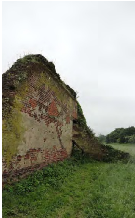
Figure 22. North Face of North Wall of Service Building showing remnants of thin cementitious render and algae caused by rainwater run-off from hard capped wall head.
