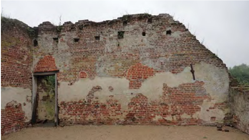
Figure 23. South Face of North Wall of Service Building showing remnants of thin lime render which has hollow sections, recently patched in areas of new handmade brick and new oak lintels, props and brickwork to doorway.
