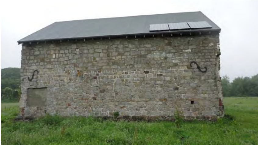
Figure 12. South Elevation of Vaulted Chamber showing photo voltaic cells on felted roof and 1920's window insertion without lintel.
