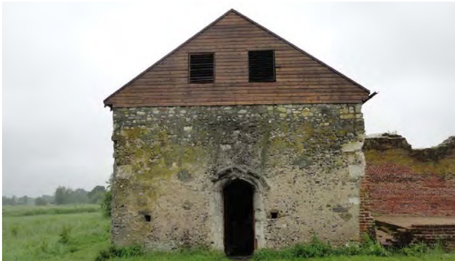
Figure 9. East Elevation of Vaulted Building showing hard cement mortar packing to upper section of elevation.
