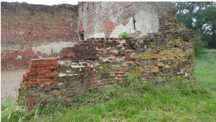
Figure 24. East Face of East Wall of Service Building showing very poor consolidation work. Varying colouration of pointing due to uncontrolled sourcing of sand and bricks to wall end with frogs exposed on upper face of bricks.
