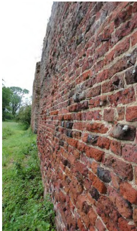
Figure 18. West face of brick wall of Service Building (former external elevation) showing extent of erosion to brick.
