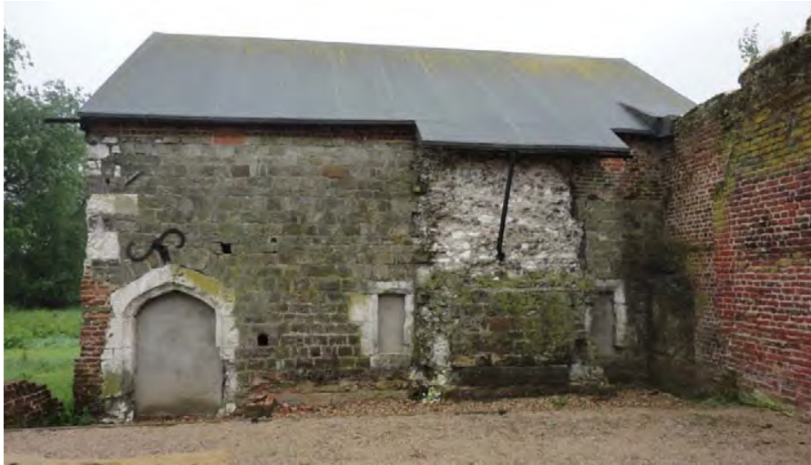
Figure 15. North Elevation of Vaulted Building showing algae growth on walls due to damaged and inadequate gutter system.
