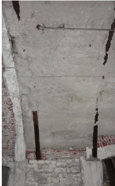
Figure 3. Circa 1920's replacement of brick to northern section of vault bay 1 and 2 with in situ concrete. Thin layer of concrete to face of rusting steel springs could detach.
