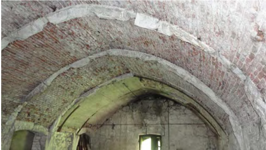
Figure 1. View of vaults looking East showing fractured chalk ribs and concrete repairs to end two bays of vault.
