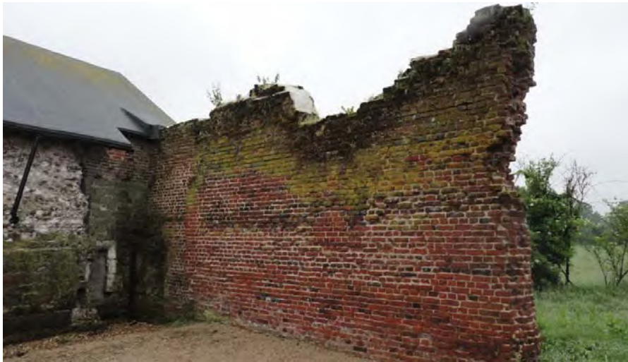
Figure 21. Southern Section East Face of Service Building West Wall showing unsightly white cement mortar capping to wall head and dampness concentrated at wall head due to rainwater run-off; poorly finished area of recent re-pointing in lime mortar.
