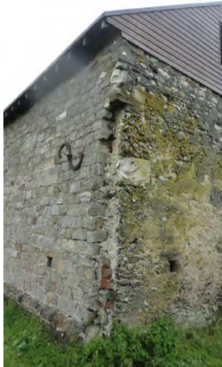
Figure 10. Missing stack of masonry from South East corner of Vaulted Building.
