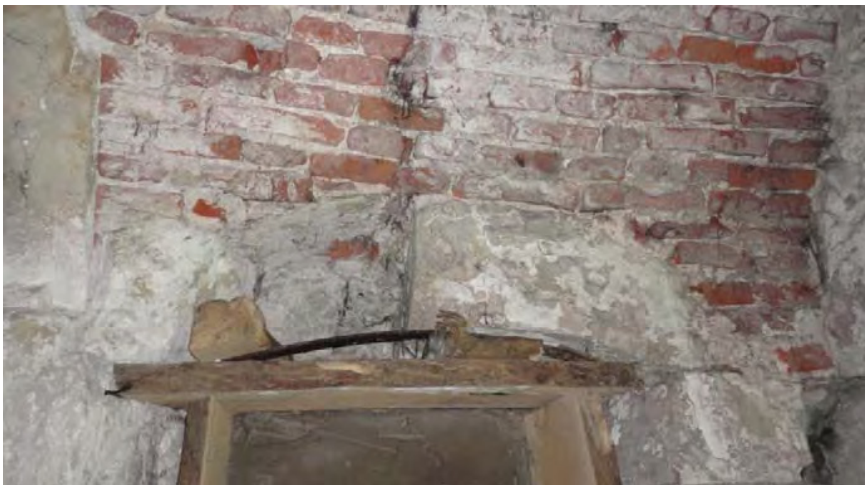
Figure 7. Iron bar supporting remaining half of chalk lintel to window in north wall of bay 5.
