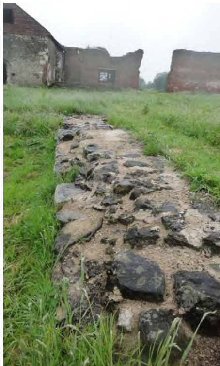
Figure 26. Low wall head remains to South End of Great Hall that have been consolidated with lime mortar that has been degraded by frost action.
