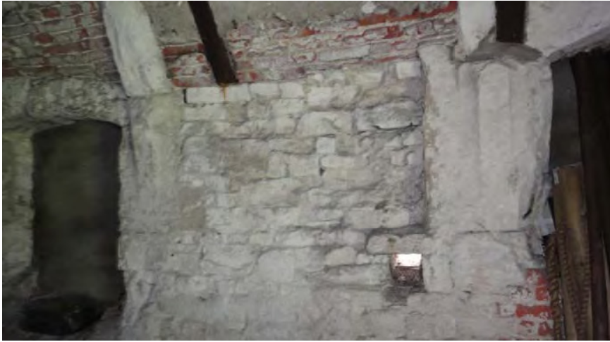
Figure 5. Good example of intact chalk spring stone and small vent opening.
