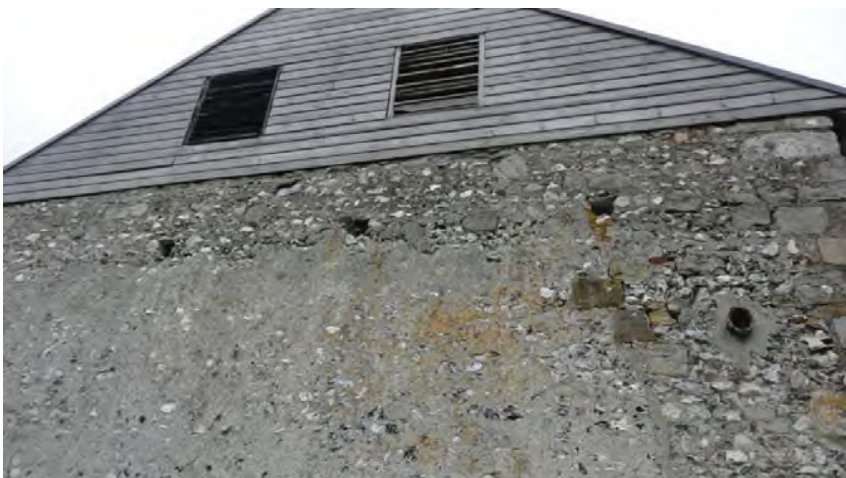
Figure 14. West Elevation of Vaulted Building showing hard sand cement mortar packing to upper section of flint walling and degrading timber louvers.
