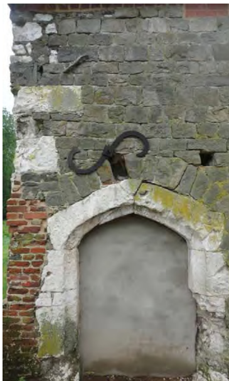
Figure 16. Cracked and settled moulded chalk door lintel on North Elevation of Vaulted Building and missing Heathstone voussoir to relieving arch.
