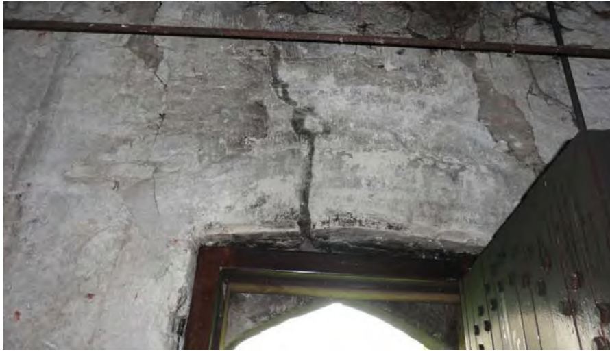
Figure 8. Previously filled cracks above door in East Elevation.
