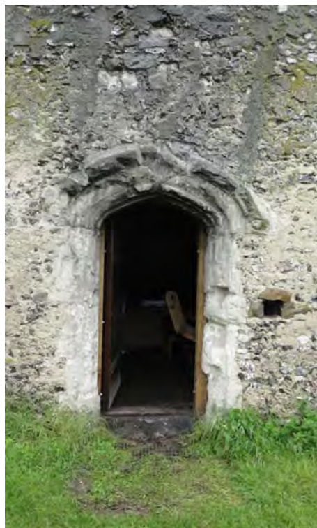
Figure 11. 15 th century moulded chalk door surround to South East Elevation with Lime Shelter Coat finish.
