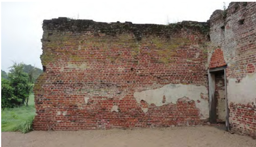
Figure 20. Norther Section East Face of Service Building West Wall showing remnants of lime plaster.
