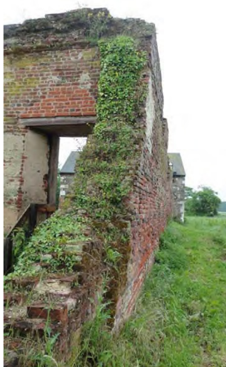
Figure 19. Consolidated wall end to West Wall of Service Building showing ivy growth which should be removed. Also recently installed timber lintels and steps to door opening.
