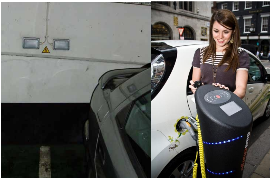
Figure 32 Electric vehicle charging points can be very low cost plug spurs (left) or dedicated kerbside points (Image © Chargemaster)
