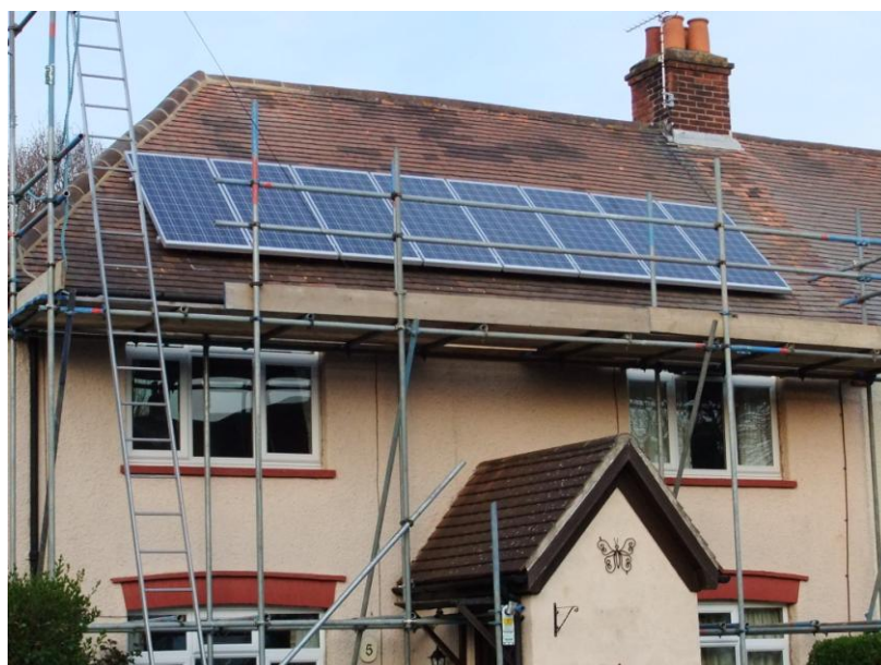
Figure 28 Private installation of PV retrofit (Kirby Road, Horsell)
