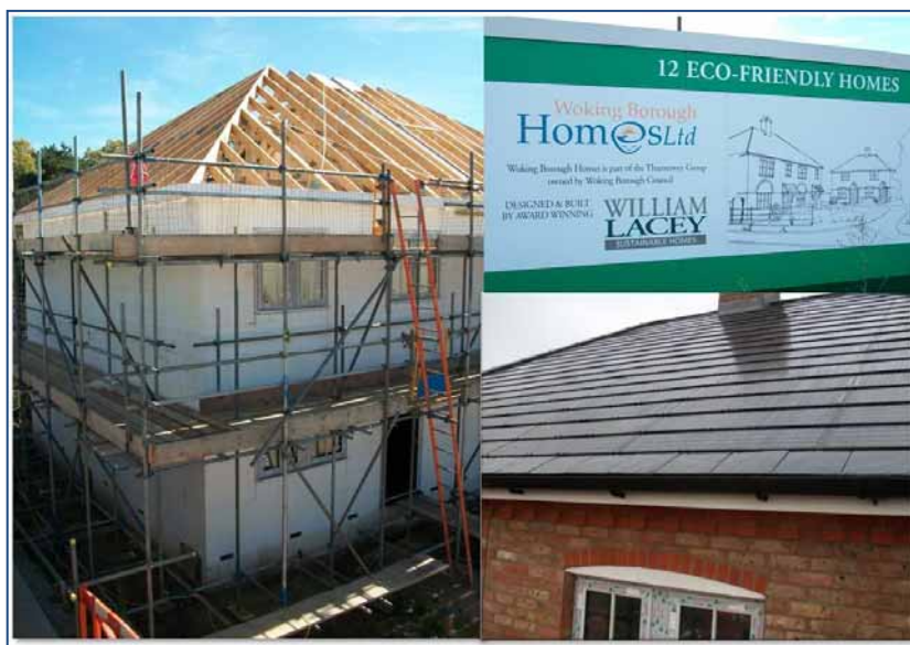
Figure 19 New Code Level 5 family homes under construction by Woking Borough Homes at Brookwood Farm, Knaphill (source: ecsc Ltd.)
