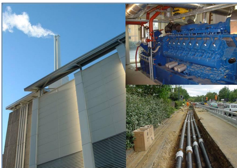
Figure 18 Woking town centre energy station provides heat, power and cooling to public buildings, commercial developments and homes in the north east sector of the town (source: ecsc Ltd.)
