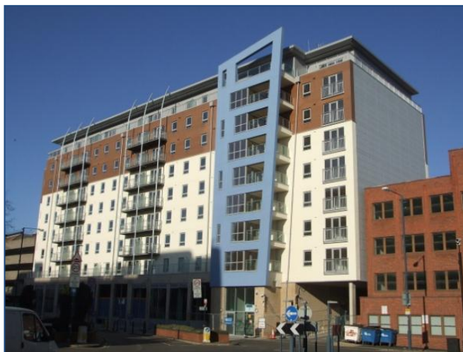
Figure 22 Enterprise Place is a development of 129 apartments in Woking town centre and was granted planning consent in 2006 subject to a legal agreement requiring connection of hot water and heating supplies to the town
