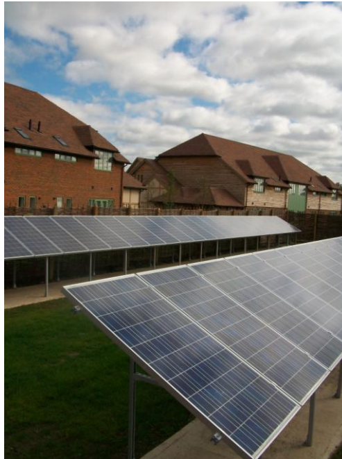
Figure 21 Retirement Village's development of 42 extra care units is in an edge of Green Belt location at Mayford. The planning consent secured very high standards of energy efficiency, along with a small CHP unit and large PV arrays that have been sensitively screened.
